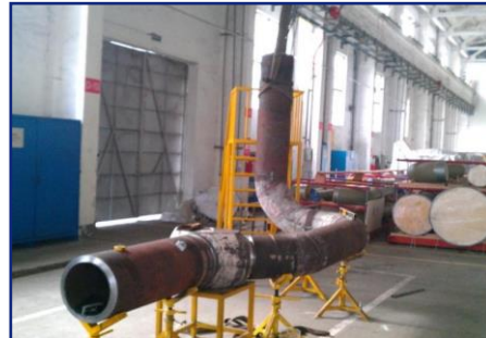
MAIN STEAM PIPING
